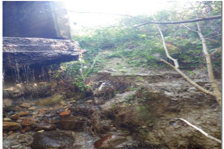
Photo 52: Unnamed Tributary 03 – Facing upstream at east side of culvert, showing collapsed embankment and erosion.
