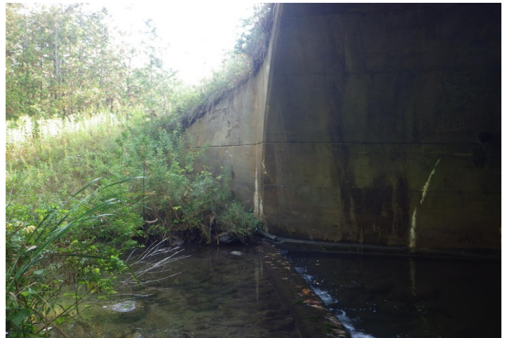
Photo 54: Unnamed Tributary 04 – Facing east at culvert, showing concrete ledge at culvert inlet.
