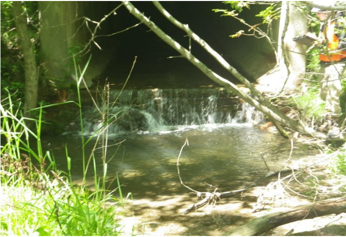
Photo 67: Unnamed Tributary 06 – Facing upstream to culvert, showing perched condition.
