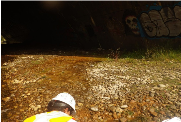
Photo 86: Shelter Valley Creek – Iron stains on east side of downstream culvert end.
