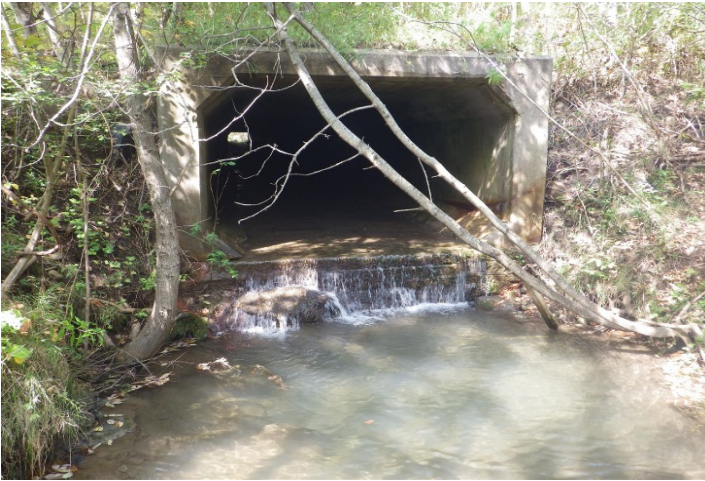
Photo 67: Unnamed Tributary 06 – Downstream culvert, facing upstream, showing perched condition.
