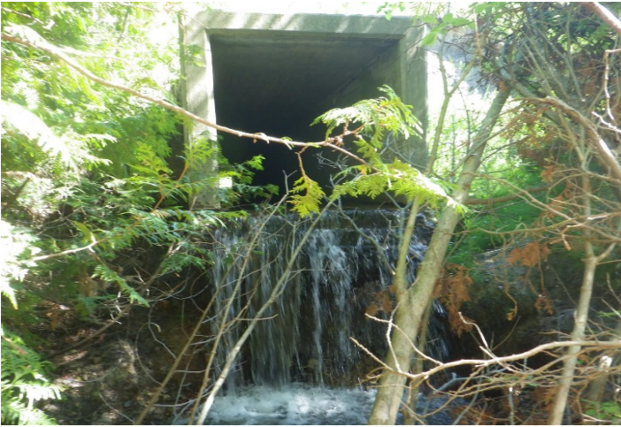
Photo 43: Unnamed Tributary 03 – Facing upstream towards perched culvert.
