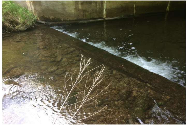
Photo 50: Unnamed Tributary 04 – Facing downstream showing concrete ledge at culvert inlet.
