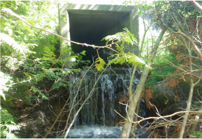
Photo 43: Unnamed Tributary 03 – Facing upstream towards perched culvert.
