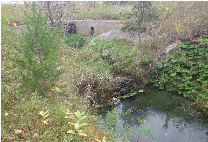
Photo 137: Unnamed Tributary 13 – Facing upstream, showing concrete apron and plunge pool.
