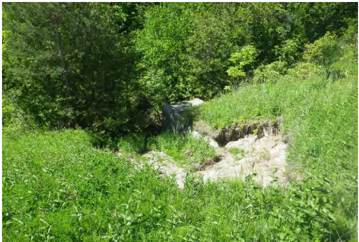
Photo 48: Unnamed Tributary 03 – Facing south from Highway towards culvert, showing collapsed embankment.
